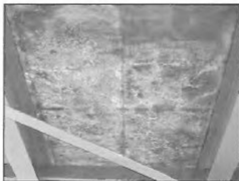
Figure B-14—Efflorescence on the Underside of the Deck in Span 1
