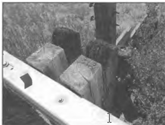
Figure B-5-Decay in Timber Rail Posts
